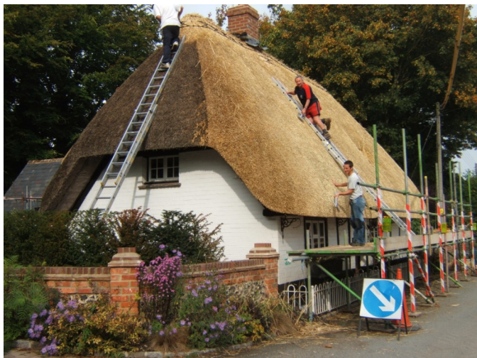
Our Master Thatcher making the thatch of a 450 year old cottage in Ablington good for another 20 to 30 years.
