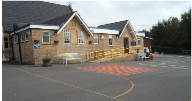
St. Michaels C of E Primary School, still recognisable after 150 years of continuous use, but in need of modernisation. The school attracts pupils from a wide area.
